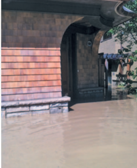
The Roxboro Glen Road home, damaged by the flood in 2013.
